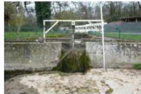
Vanne A + atterrissement
